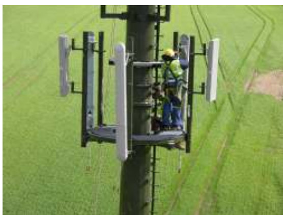
DeaCom engineers at work
